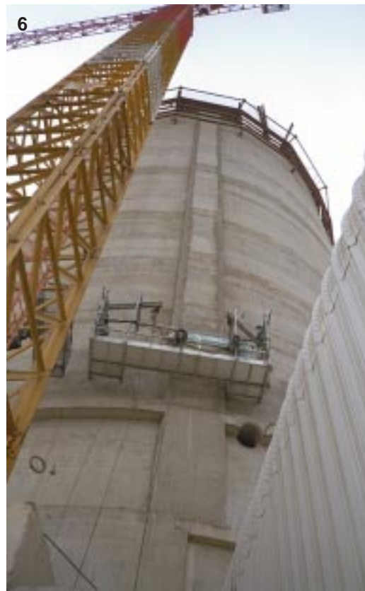
6 - Special platform for prestressing concrete (Nuclear power stations, cement silos, liquid gas tanks, bridges, viaducts, etc. . .). Operated by hydraulic TIRFOR TU-16H or TU-32H lifting machines and fitted with mobile beams for handling the prestressing rams.
