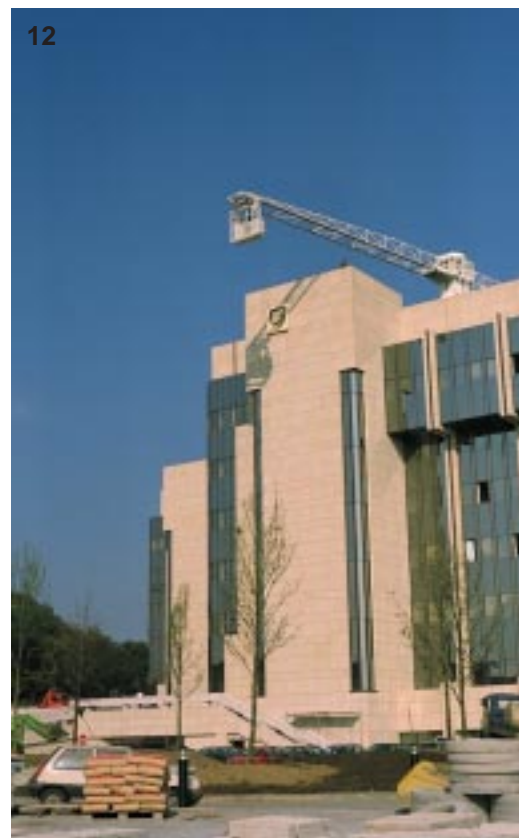
12 - Special Building Maintenance Unit (BMU). (Luxembourg International Bank). All the traversing and rotating manoeuvres are controlled and carried out by programmable logic control (PLC) which takes the machine with its cradle automatically to the working area selected before leaving the parked area.
